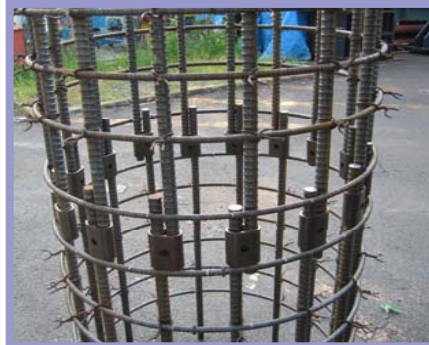
Rebar-Cage for Cast-in-place concrete pile
