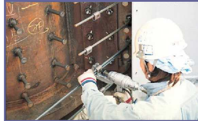
Reinforcements for SRC beam-Column joint
