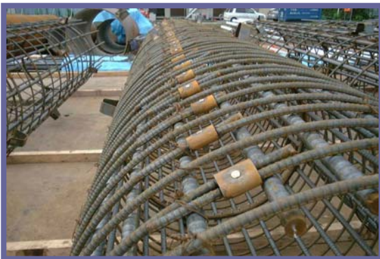
Rebar-Cage for Cast-in-place concrete pile
