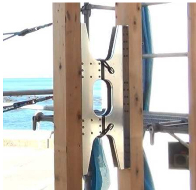
(f)裏面も同手順で施工
