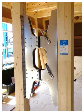
(f)裏面も同手順で施工
