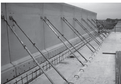
橋梁の高欄部型枠
