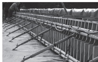
橋梁の高欄部型枠
