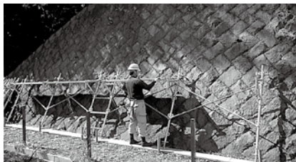
② Installation of horizontal steel plates
