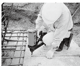
(1) Fix Bottom runners (No.4) on the concrete with nails.
