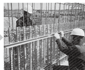
(3) Pass separators through Washers(No.7) ->panels (No.1) and battens (No.2,3) and tighten Nuts(No.6) from outside.
