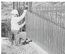
(4) Set the other side of panels (No.1) and fix them temporarily.
