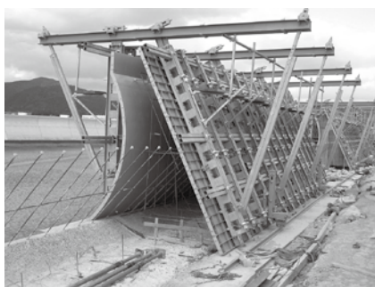
Wave breaker upper formwork
