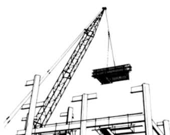
④ Lifting and installing H-beam Scaffolding hanging frame
