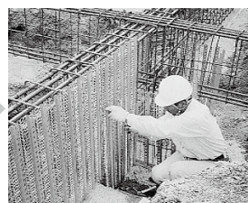
(2) Connect/Bend panels (No.1) and set them at the proper location.
