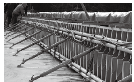
Formwork for bridge parapet
