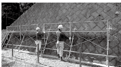
③ Installation of extendable handrails
