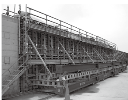
Inverted T retaining wall
