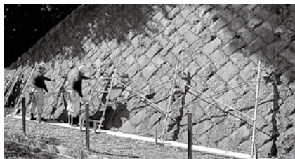
① Installation of slope stanchions
