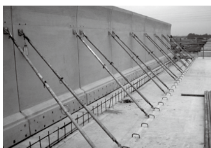
Formwork for bridge parapet
